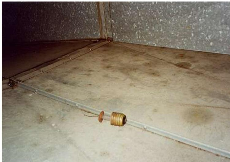
**Picture 4: Duct with a dust layer of 25 g/m<sup>2</sup> (low standard)**
