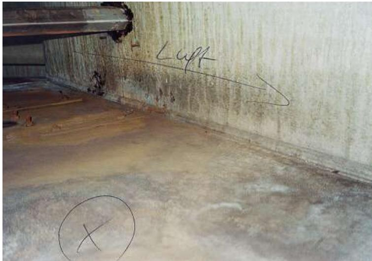
**Picture 5: Duct section behind a humidifier**
