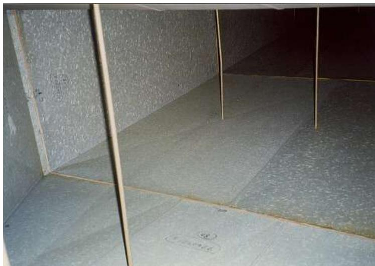
**Picture 2: Duct with a dust layer of 5 g/m<sup>2</sup> (high standard)**
