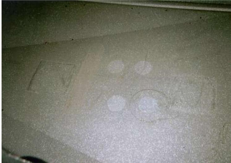
**Picture 3: Duct with a dust layer of 10 g/m<sup>2</sup> (medium standard)**
